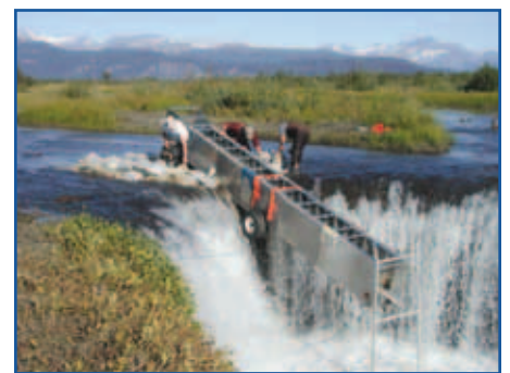
The crew at Cannery Creek uses sand bags to help divert water through the steppass.
