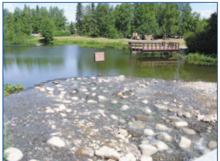
The finished roughened channel allows fish to move easily to the lake.
