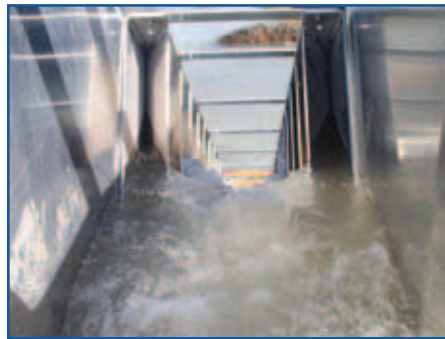
The baffle design of the steeppass slows the velocity of the water to allow fish to swim easily up the incline.
