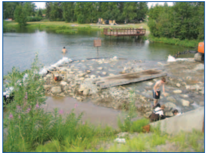
Construction crews used rock and gravel to create a natural channel.
