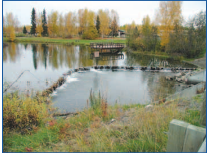
The dam structure made migration of fry to the lake nearly impossible.
