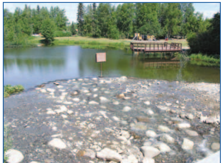
The finished roughened channel allows fish to move easily to the lake.
