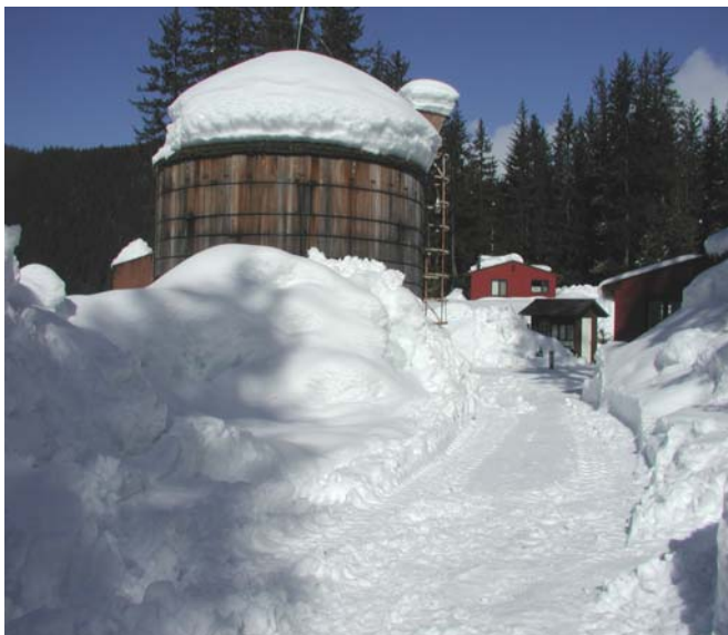
One of the many elements the crew has to contend with at Tutka Bay Hatchery is the annual snow fall. Pictured above is the water settling tower blanketed by an eight foot snow load in mid April of 2002.
