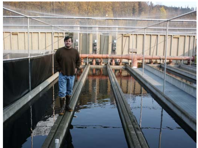
Robert Blankenship, the new Trail Lakes Hatchery manager, surveys the outdoor raceways. The bird netting that now covers these raceways was one of the many changes implemented by the hatchery crew to increase production through proper sanitation.
