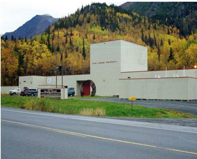
Trail Lakes Hatchery underwent a major facelift this past year. The exterior of the building received a new coat of paint, and the roof had numerous repairs due to the aging process. The process water wells were redeveloped to allow for future uninterrupted flows for fish development.
